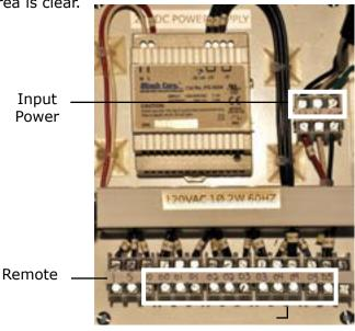
Input Power Terminals - The incoming power terminals are located on the right side of the sub panel mounted in the back of the timer box. Voltage should be 100-240 volts AC, 50/60 Hz. (The power supply adjusts to the delivered input power and provides 24 volts DC to the timer circuits.)
